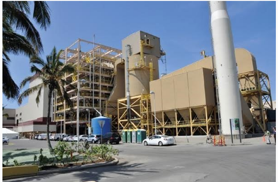
The City's H-Power waste-to-energy plant in Campbell Industrial Park.
